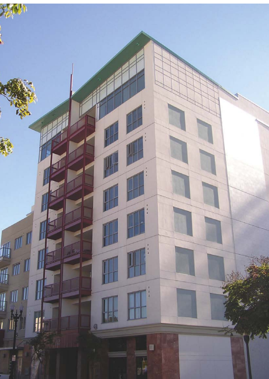
Painted galvanized steel was used for Nexus' balconies.
