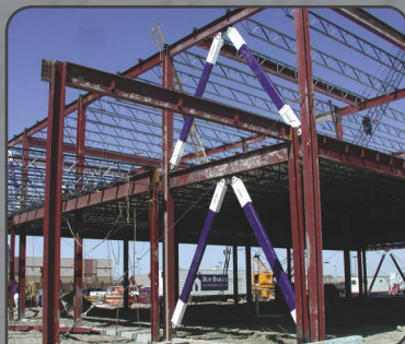
STAR SEISMIC POWERCAT Pinned connections
