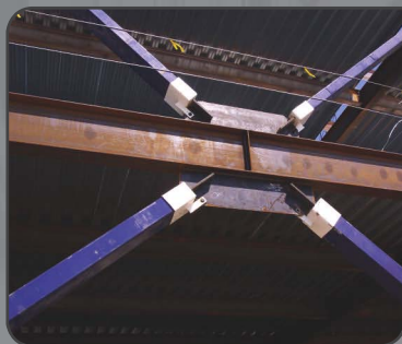
STAR SEISMIC WILDCAT Welded connections
