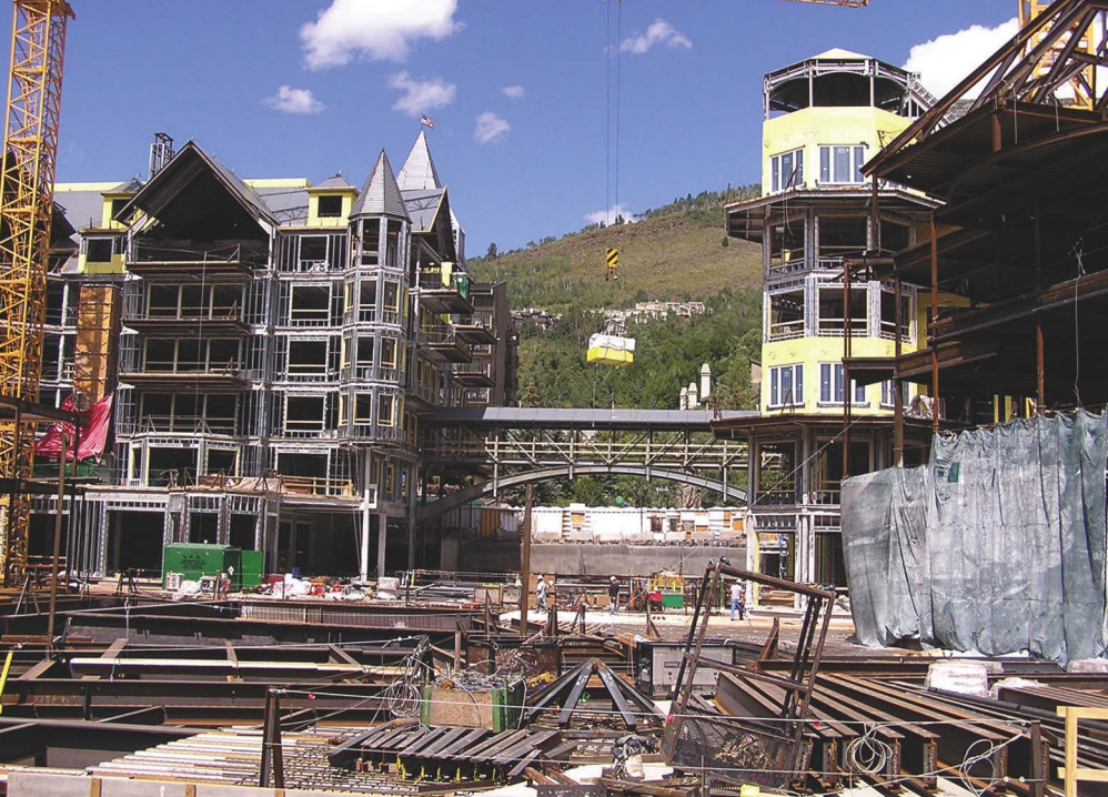
An 85-ft pedestrian bridge connects the east and west areas of the Arrabelle development. The entire project had more than 500 steel beam penetrations.
