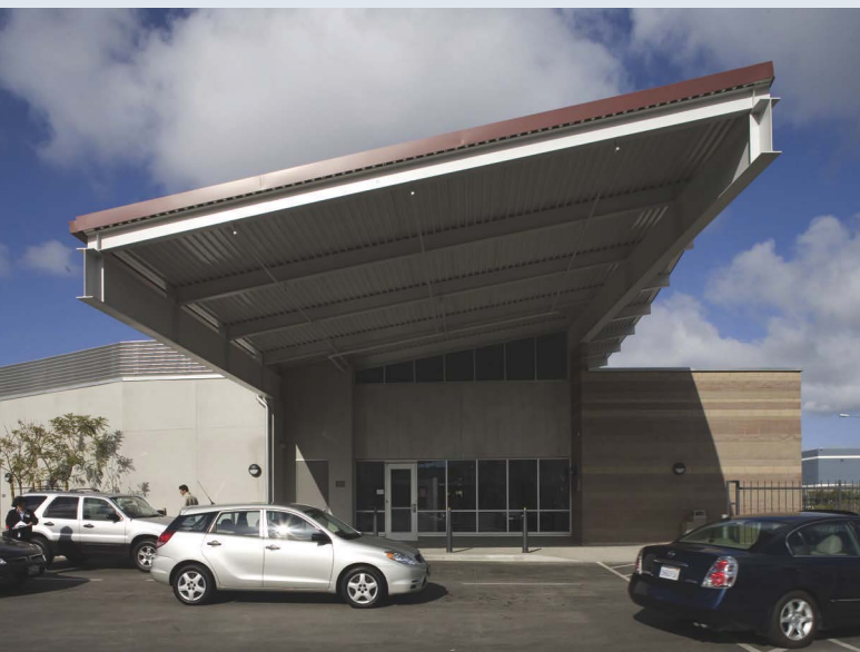
Exposed metal roof deck in a Department of Motor Vehicles facility in southern California (see "Getting the Green Light," January 2008).
